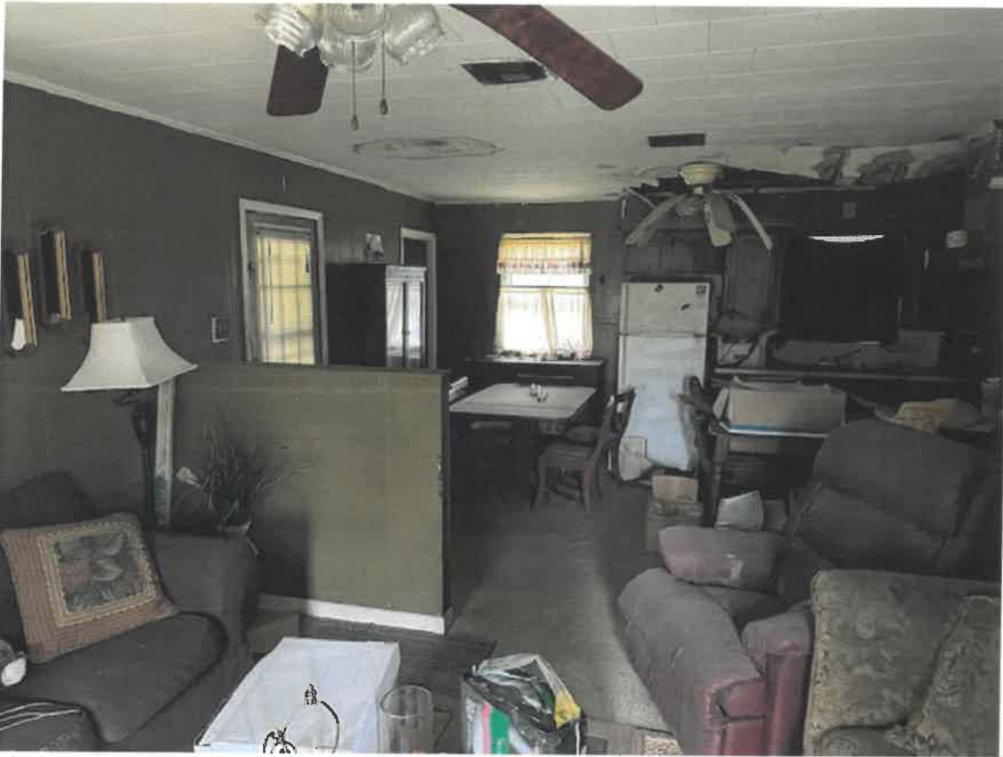
Picture taken March 27, 2025: Picture of dwelling while entering front door. Home appears to be abandoned due to structural roofing damage from fallen tree.
