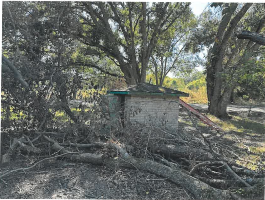
Picture taken November 15, 2024: Property has large piles of downed trees causing blighting and creating habitat for pests and vermin, accessory structure is not maintained.
