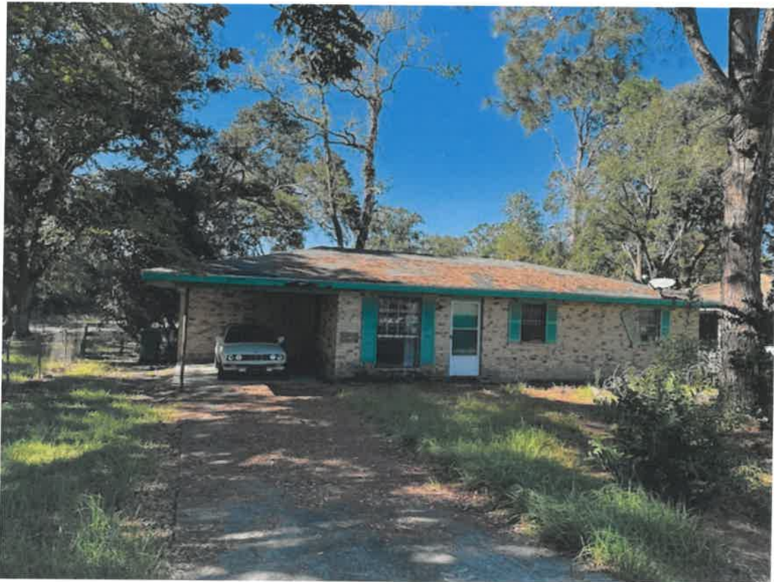
Picture taken November 15, 2024: Front view of property, overgrown with foliage causing blighting.
